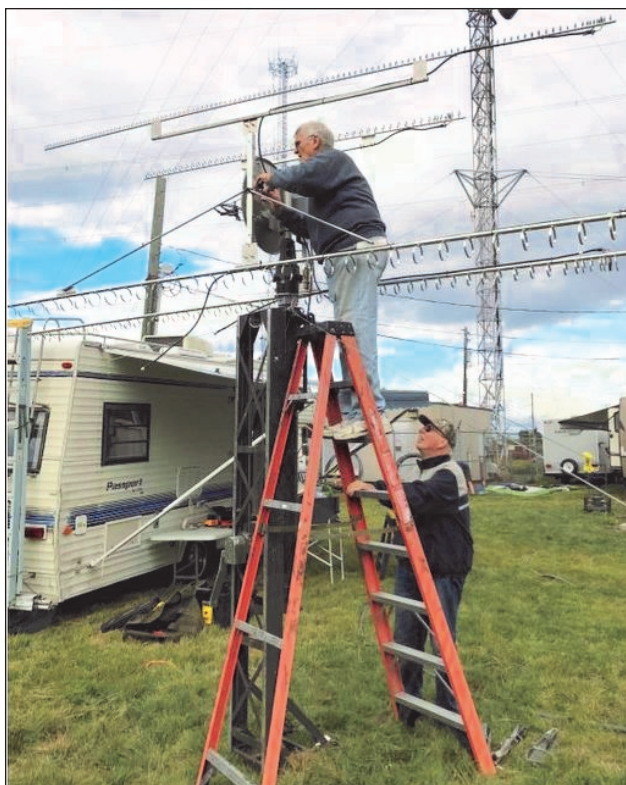
Ray N3RG and Bob W2SJ putting the final touches on the Microwave stack before raising the tower on High Knob, 2017
